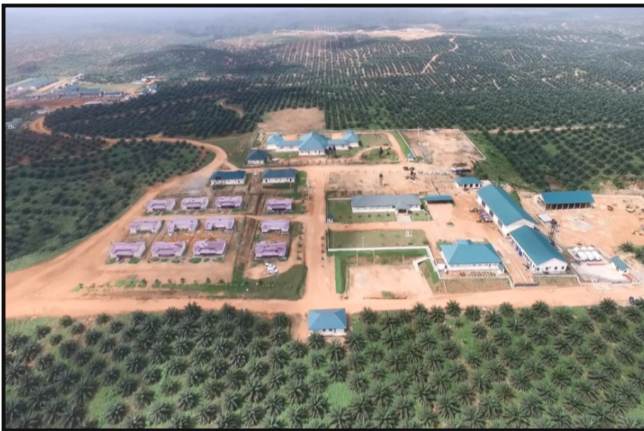
Aerial view of Calaro Estate
